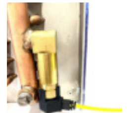
Figure 6: Clip + Sensor Installed
