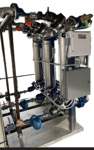
"What made the Thermo-Pack a good fit, was first the size. We want to be able to convert building steam laterals to hot water by putting these in a vault, with the controls in the building," stated Frank Perry. The vertical packaged skid was customized to easily fit within the restraints of the mechanical room.
